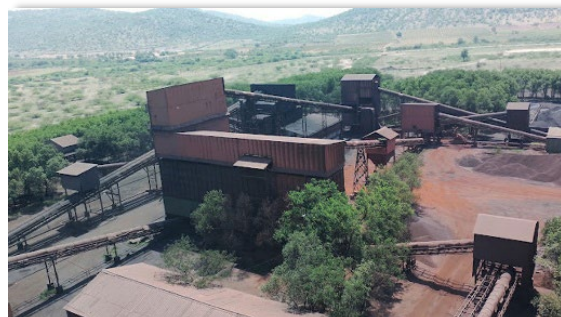
Ananthapur Unit-II, Andhra Pradesh
